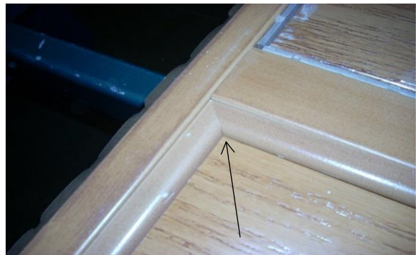
Figure 4 Miters should be tight
