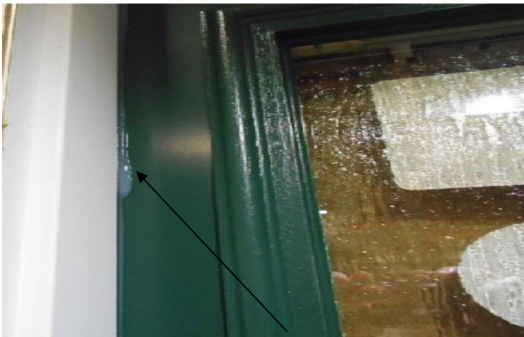
Figure 9 Clean up caulk squeeze out
