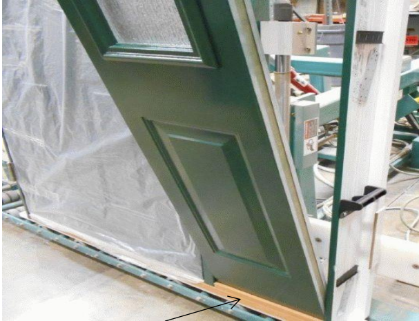
Figure 7 Insert the bottom of the sash first
