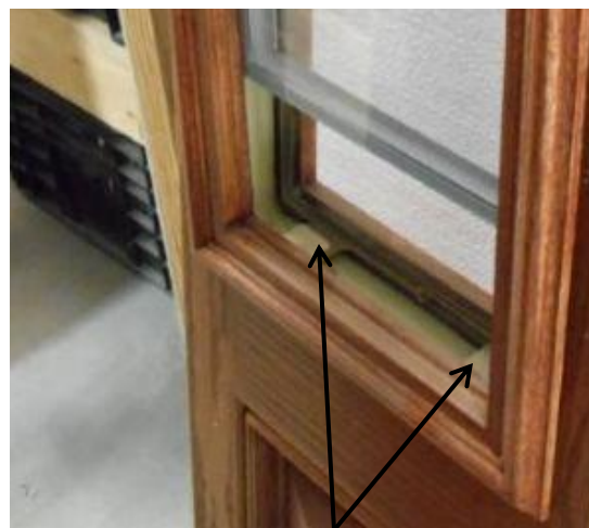
Figure 9 Glass should be seated on tabs
