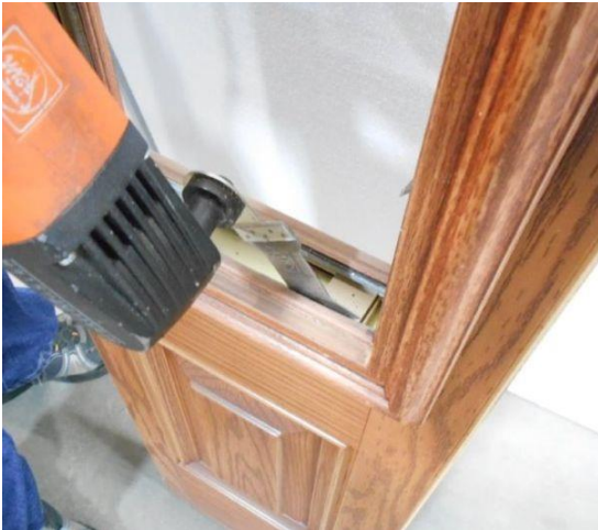
Figure 3 Cut the bottom tabs
