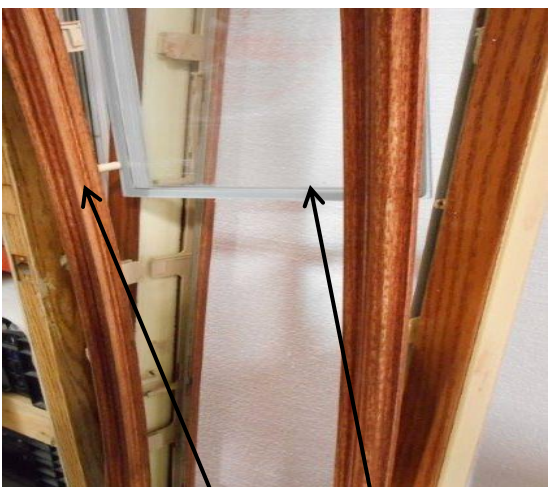
Figure 8 Pull back frame and slide glass into place
