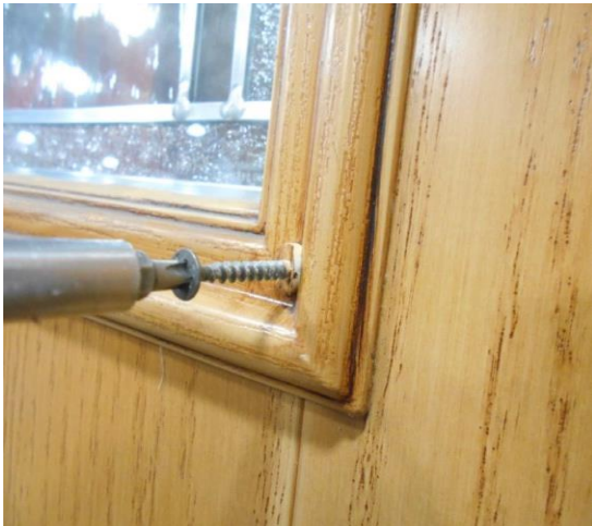
Figure 1 Remove screw plugs
