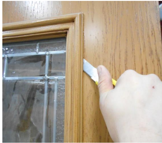
Figure 4 Cut caulk between frames and door
