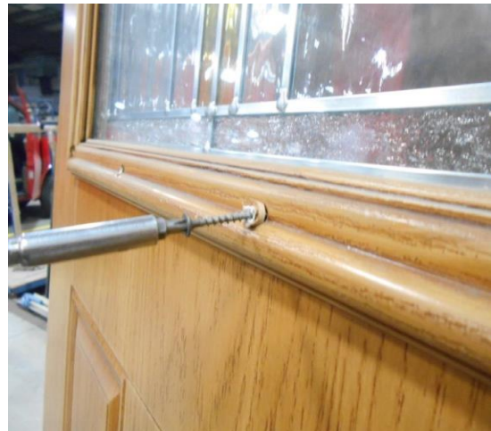
Figure 2 Remove screw plugs
