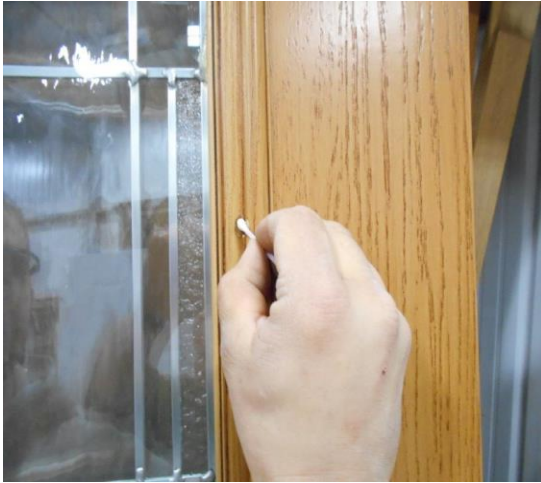
Figure 11 Apply touch up to screw plug
