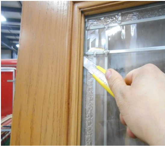
Figure 3 Cut caulk between frames and glass
